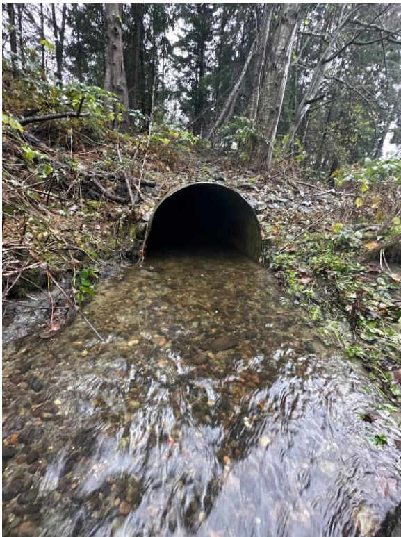
Figure 2-8: Outlet of Queensborough Creek under SR 527
