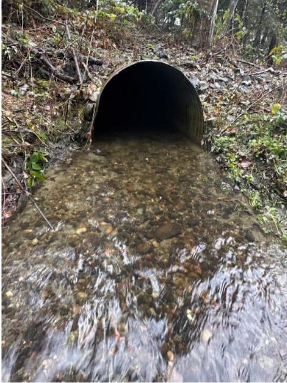
Figure 2-12: Sediment at SR 527 outlet
