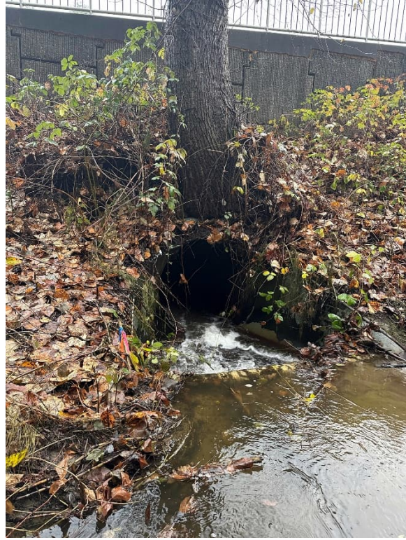
Figure 2-7: Inlet of Queensborough Creek under SR 527
