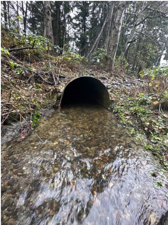
Figure 2-8: Outlet of Queensborough Creek under SR 527
