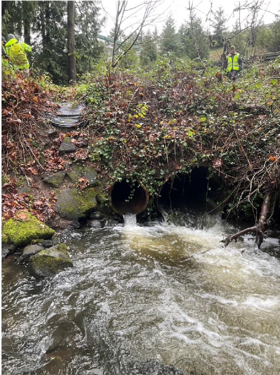
Figure 5 Property Access Culverts Downstream of Juanita Creek I-405 MP 21.94
