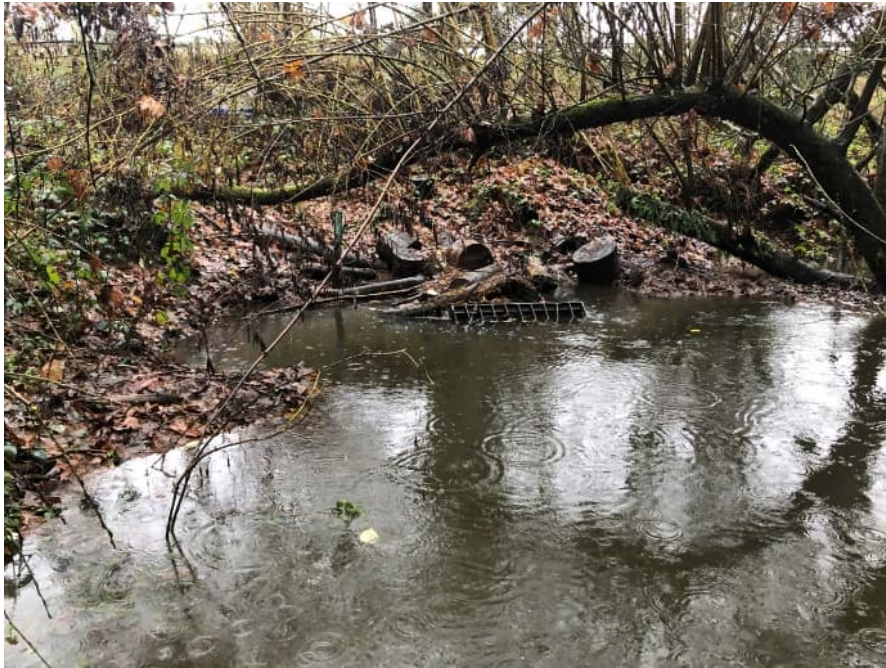
Figure 3 Juanita Creek I-405 MP 21.94 Existing Culvert Inlet
