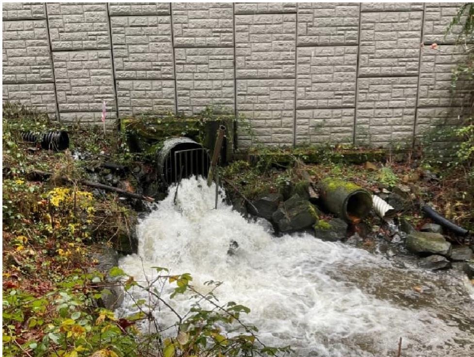
Figure 4 Juanita Creek I-405 MP 21.94 Existing Culvert Outlet
