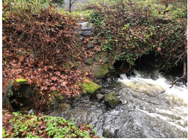
Figure 2-4: Culvert downstream of the I-405 crossing
